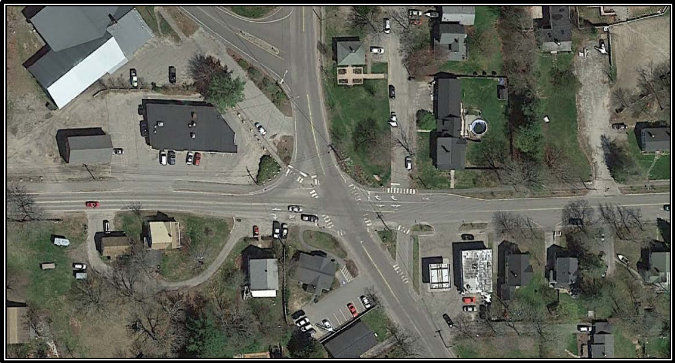
Figure 9: Site #5 - "Five Corners" Intersection
